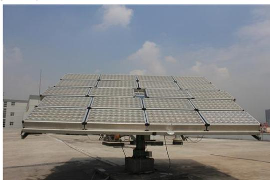
Fig.1. A 5kW HCPV with solar tracking system
