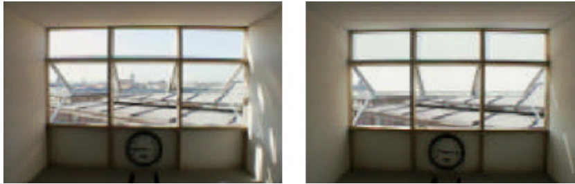
Fig.5- thermotropic polymer laminate glasses be applied as overhanging shelves on the outside
