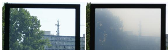
Fig.2- Thermochromic window with semi-opaque view to outside
