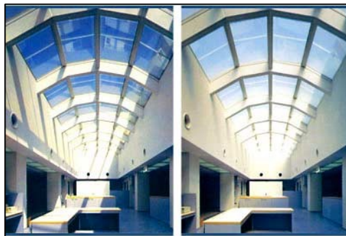
Fig. 6: Two manners of liquid crystal windows [10]
