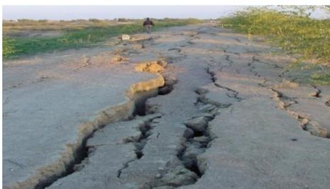
Figure 12. Cracking and inelastic deformations of the crest embankment was caused by the 2001 Bhuj earthquake in India. The prediction of cracks and damage requires nonlinear dynamic analyses and modelling of dam materials. Sort by[19].
